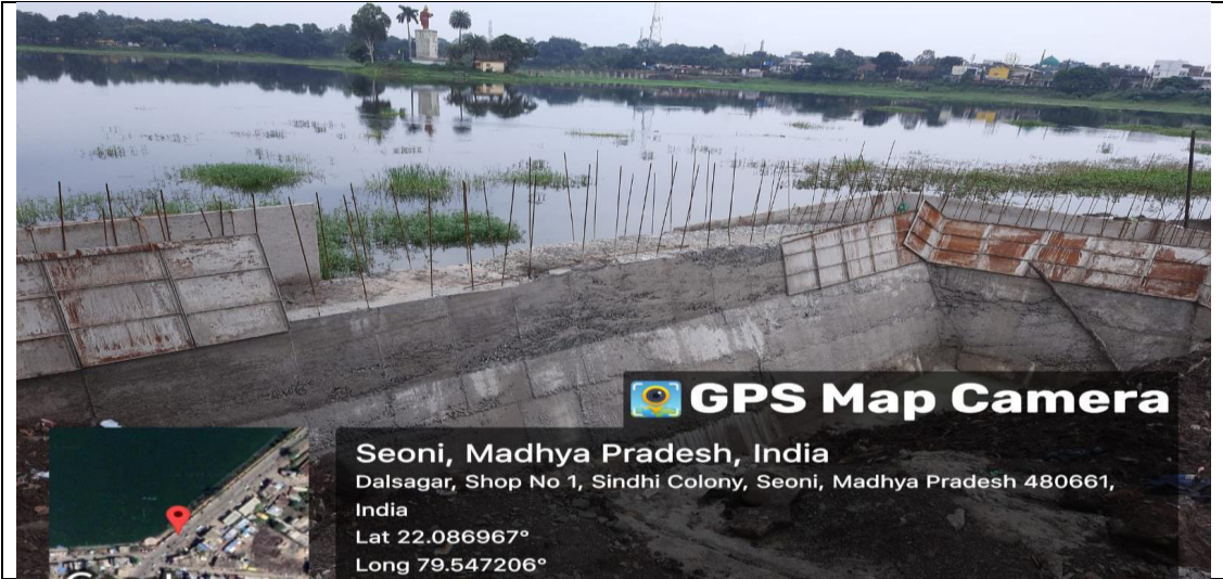
Construction of retaining wall inside the lake submergence
