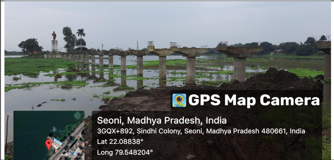
Construction site of Dal SAGR Lake
